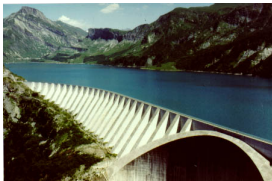
Cornet de Roselend dam (France)
