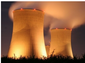
Cattenom nuclear power plant (France)
